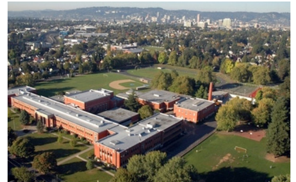
Site & Context, Present Day
